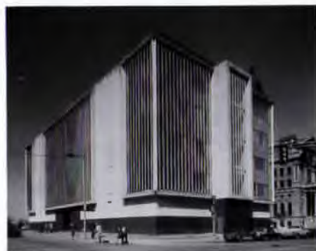
The 1958 Tarrant County Civil Courts Building, ABOVE, has been transformed by artist Richard Haas and architects George C.T. Woo and Partners into a visually conformist Courthouse neighbor, LEFT. Just blocks away, the spire-capped Tarrant County Courts Facility, BELOW LEFT, and the more modest Tandy Technology Center, BOTTOM LEFT, add to the visual complexity of northern downtown's urban fabric.
