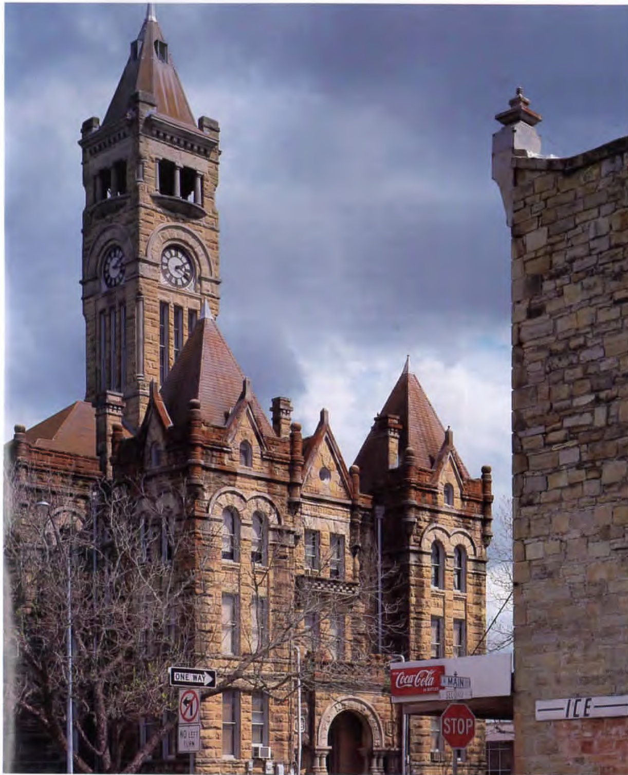
Grimes County Courthouse in Anderson, FACING PAGE, sits athwart the main axis of the town, rather than on a central block nestled between four surrounding streets, like the Lavaca County Courthouse in Hallettsville, ABOVE.
