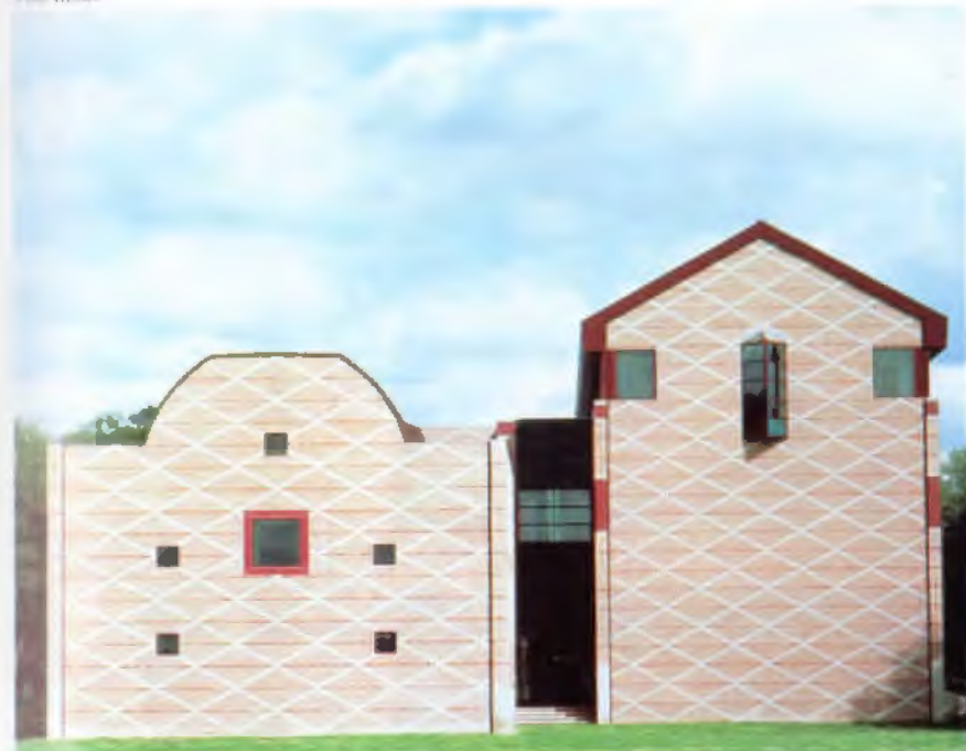
ABOVE and BELOW, RIGHT: Herring Hall, Rice University, Houston, by Cesar Pelli & Associates
