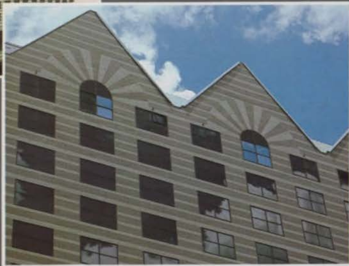
Morris+Aubry Architects. Wyndham Hotel Greenspoint, Houston. Trammell Crow Hotel Company, developers.
