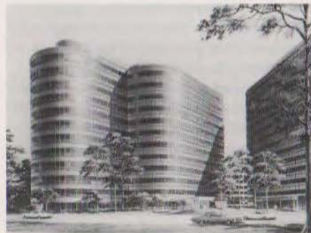
ABOVE: Design for Brookhollow Central III, Houston, developed by PIC Realty Corp. and scheduled for completion in August. Judged as the best example of energy-conscious design in the third annual energy management competition of the Houston Chapter of ASHRAE. Uses high-performance coated glass and panels of mineral asbestos, instead of aluminum. Average wall has thermal U-value of .30.
