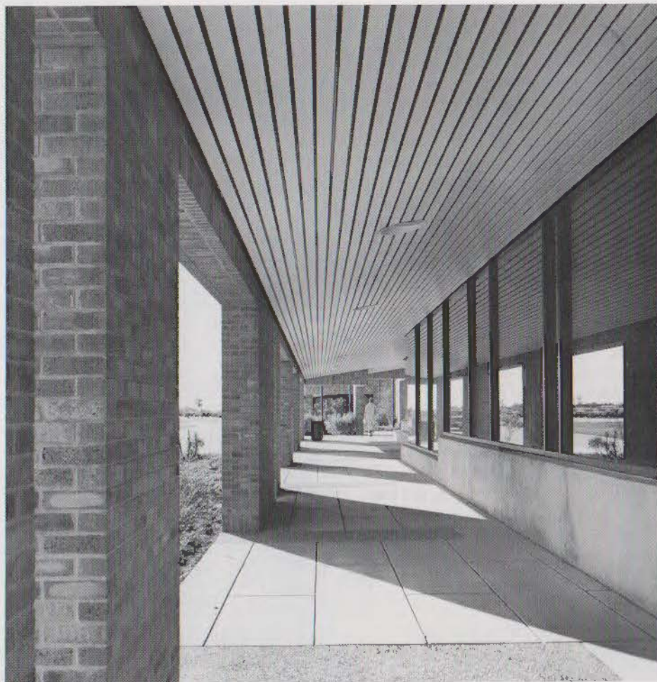
Loggia with metal-plank ceiling.
