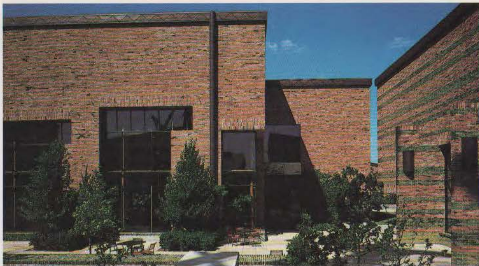
Details of glazed and plain walls at Brookhaven College.
