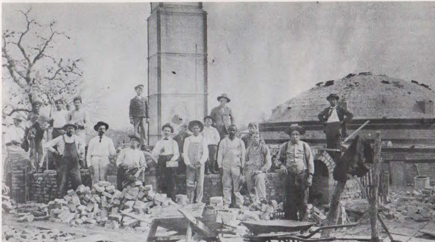
Building beehive kiln in Elmendorf, near San Antonio, before 1900.
