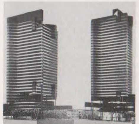
ABOVE: City Center, Fort Worth, for Bass Brothers Enterprises, Inc., by 3D/I in association with Paul Rudolph, the design architect. Includes 35- and 40-story office towers scheduled for completion in 1983. Sheathed in clear glass with reflective coating. Unique corner offices extend beyond the basically square outline in pinwheel fashion, providing windows on three sides in some offices. Metal-clad column clusters extend five to seven stories above ground.
