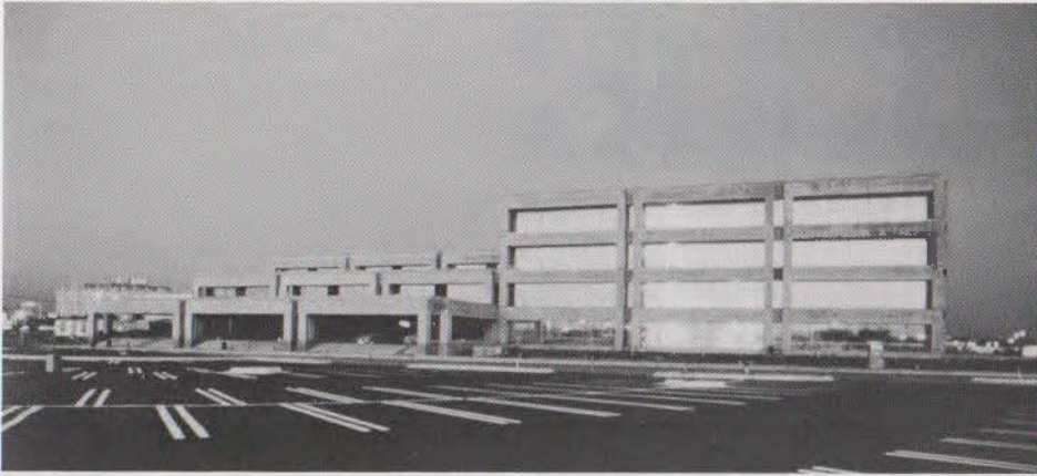
LEFT: Blue Cross-Blue Shield of Texas, corporate headquarters, Richardson, nearing completion. Sixty-ton U-shaped bents, combining two columns and one beam in a single cast, form the major structural and architectural element and provide for long spans. BELOW: Citizens Bank Center, Richardson, 1974. Bold form is achieved with 105-foot-long precast girders which provide column-free space and uninterrupted vistas on each floor.
