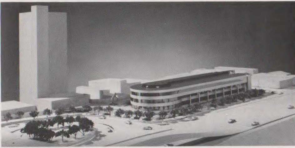
LEFT: Alfa Industries Division office building, Monterrey, to be completed this year. Horizontal banding and massing of reflective glass and aluminum panels express the dynamic lateral movement of surrounding site conditions. BELOW LEFT: Natural Gas Pipeline Co. Tower, Houston, for Gerald D. Hines as part of his Lake on Post Oak development. Sheathed in bronze glass and aluminum. Column-free corner offices overlook lakes below.
