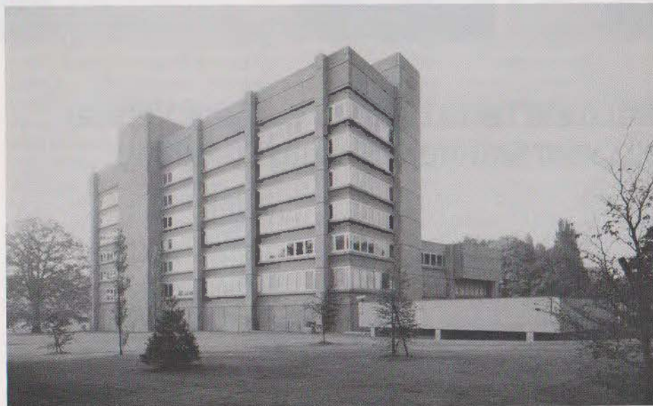
U.S. Mission, Geneva, Switzerland, 1980. Load-bearing structural elements were combined with insulation and a finely detailed skin and erected as single components. Erection of the shell, with windows, took only ten weeks.
