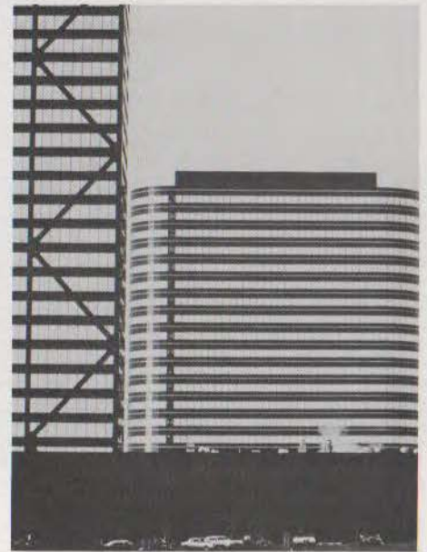
BELOW: TownCenter phase II, Southfield, Michigan, for PIC Realty Corp., designed to complement phase I tower in foreground. Gold insulating glass occupies approximately 35 percent of the surface area. A bold accent stripe, laid into a recess within the metal panels, wraps horizontally around each floor.
