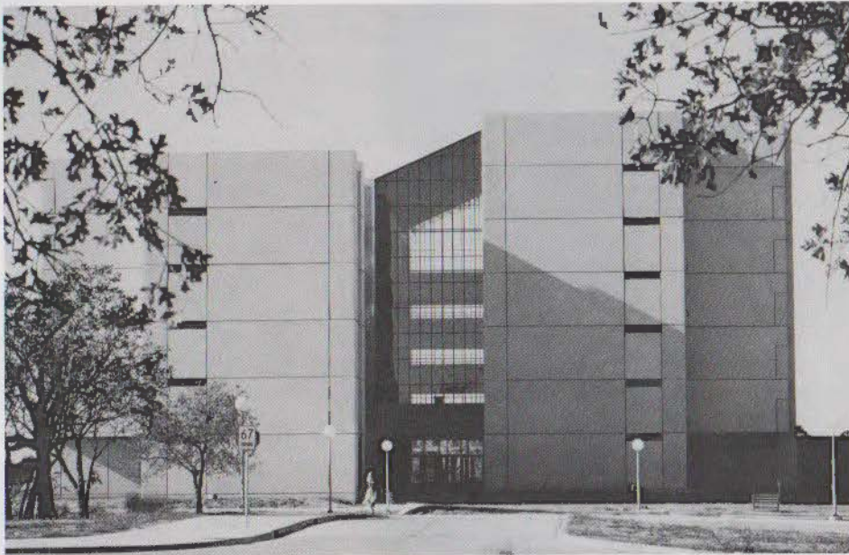
Texas A&M University Soil and Crop Sciences and Entomology Center, 1977. Structural, architectural and mechanical needs are served simultaneously by the precast building components.
