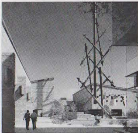
Plaza and windmill structure.
