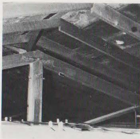
LEFT: One of the wooden trusses which carry the gallery level of the Calvert Cotton Blossom. Note metal straps on truss, original electrical supply, and hanging rod in lower right-hand corner. BELOW: Axonometric of Smith-Welch Library in Hearne.
