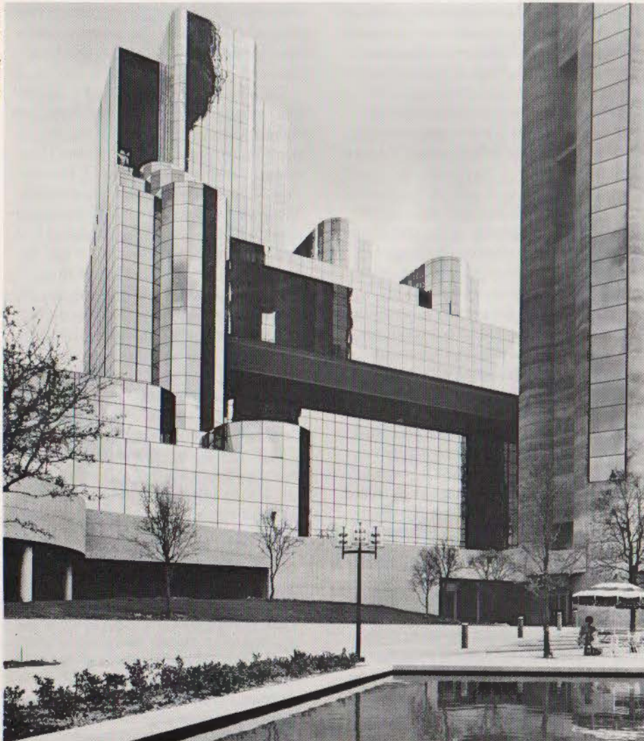
South approach by reflecting pool.
