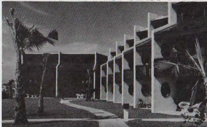
Suntides I, a 30-unit luxury condominium complex on South Padre Island, Texas, was built of concrete blocks and SUREWALL® Surface Bonding Cement to withstand high velocity winds from the Gulf of Mexico. The architect on the project was Rick Labunski.
