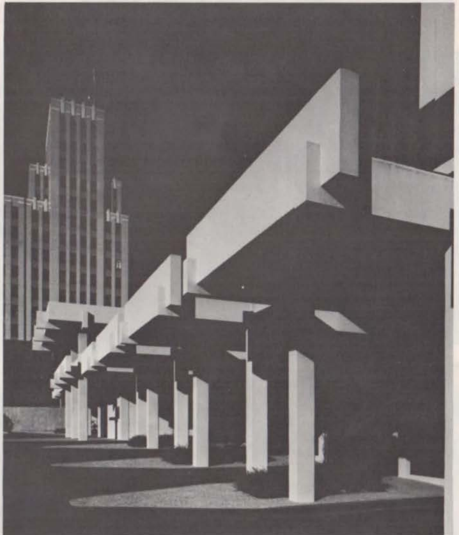
PEOPLES NATIONAL MOTOR BANK tyler, texas e. davis wilcox associates
