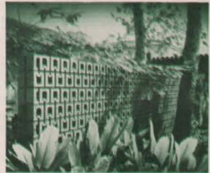
Attractive concrete block sight screen encloses patio for breezy seclusion
