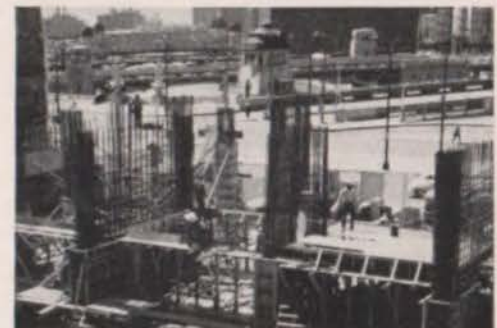
Four concrete shear walls extending across the width of the building provide necessary resistance to wind forces.
