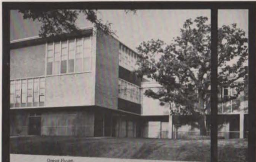
Gregg House, Austin Feltz & Granger, Architects, Austin
