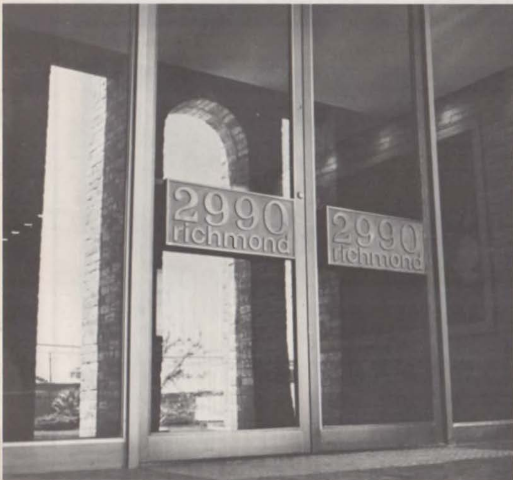
Full height doors emphasize entrance to elevator lobby.
