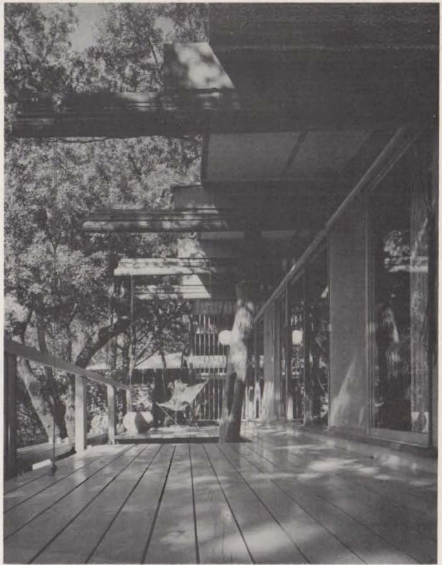
The simple structural system of post and beam is developed to provide its own rhythmic and geometric order in contrast to the irregular curves of the treetops.
