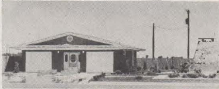
ABOVE—Above ground entrance to the new underground residence and fallout shelter in Plainview, Texas.
