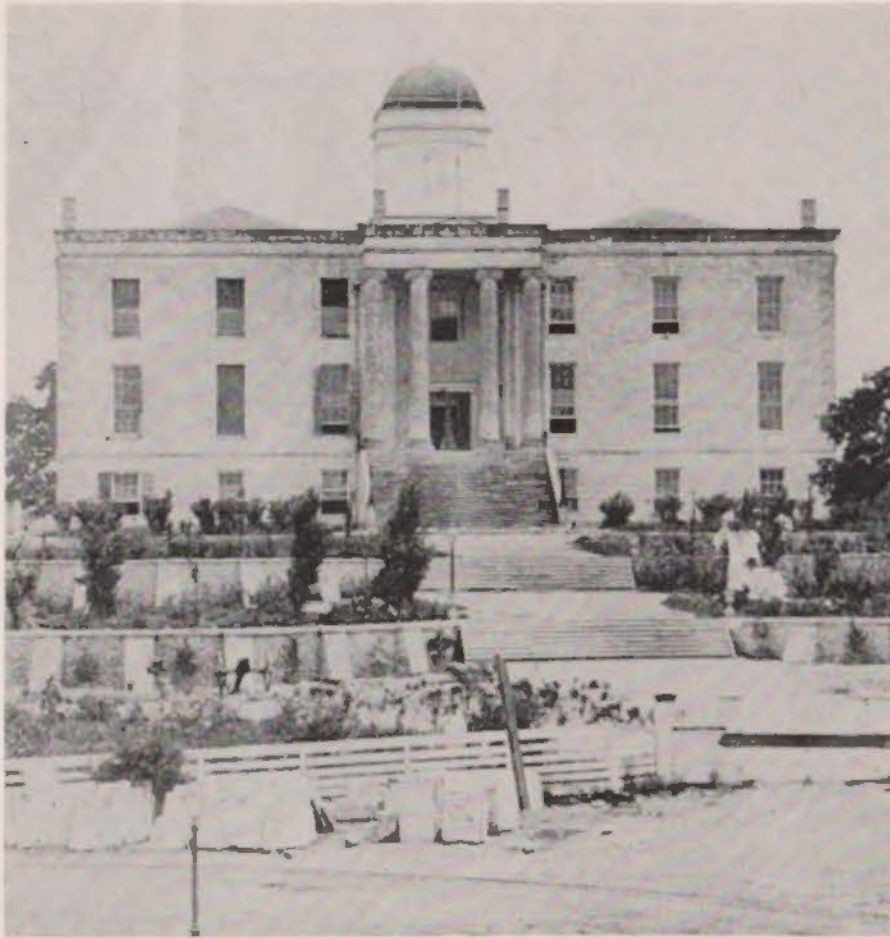
Construction of the present State Capitol was speeded up when fire destroyed the old one, shown above, which was described by this 1881 newspaperman as "the architectural monstrosity" at the head of Congress Avenue.
