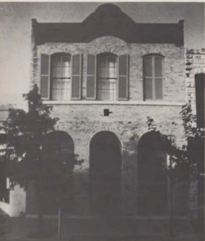
TWO OF THE THIRTY STRUCTURES to be incorporated into the proposed Historic Buildings Trail. In every case, the buildings would take on a specific function either private or public. On the left, a commercial structure converted to a townhouse and below, a residence which has become an attorney's office.
