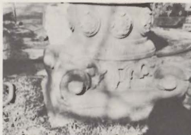
Details of column from 1890 courthouse
