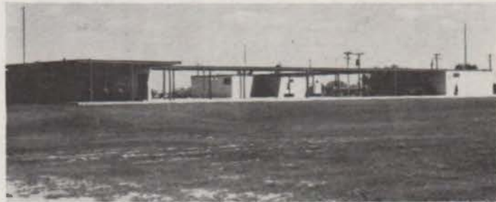
ABOVE — Above ground entrance to the new underground school and fallout shelter in Artesia, New Mexico.
