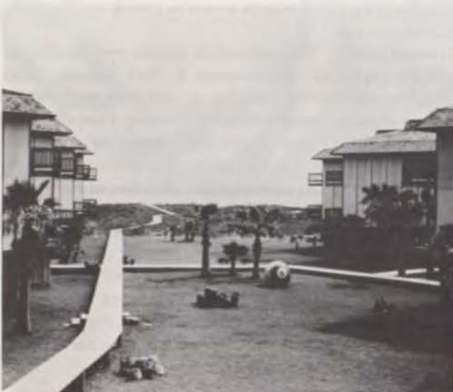
Existing condominium built to acceptable standards for the harsh weather conditions. (Living areas raised on heavy pole columns which are continued to the roof, built behind the dune line to make use of the dunes as protective wind and water barriers, use of board walks to remove destructive pedestrian traffic from the valuable dunes.) This project received minimum damage during the storm.
