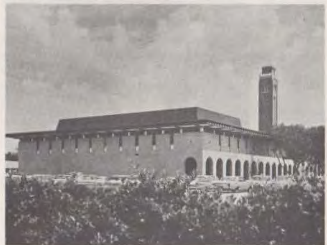
Ryon Engineering Laboratory, Rice University Wirtz, Calhoun, Tungate & Jackson, A.I.A., Architects
