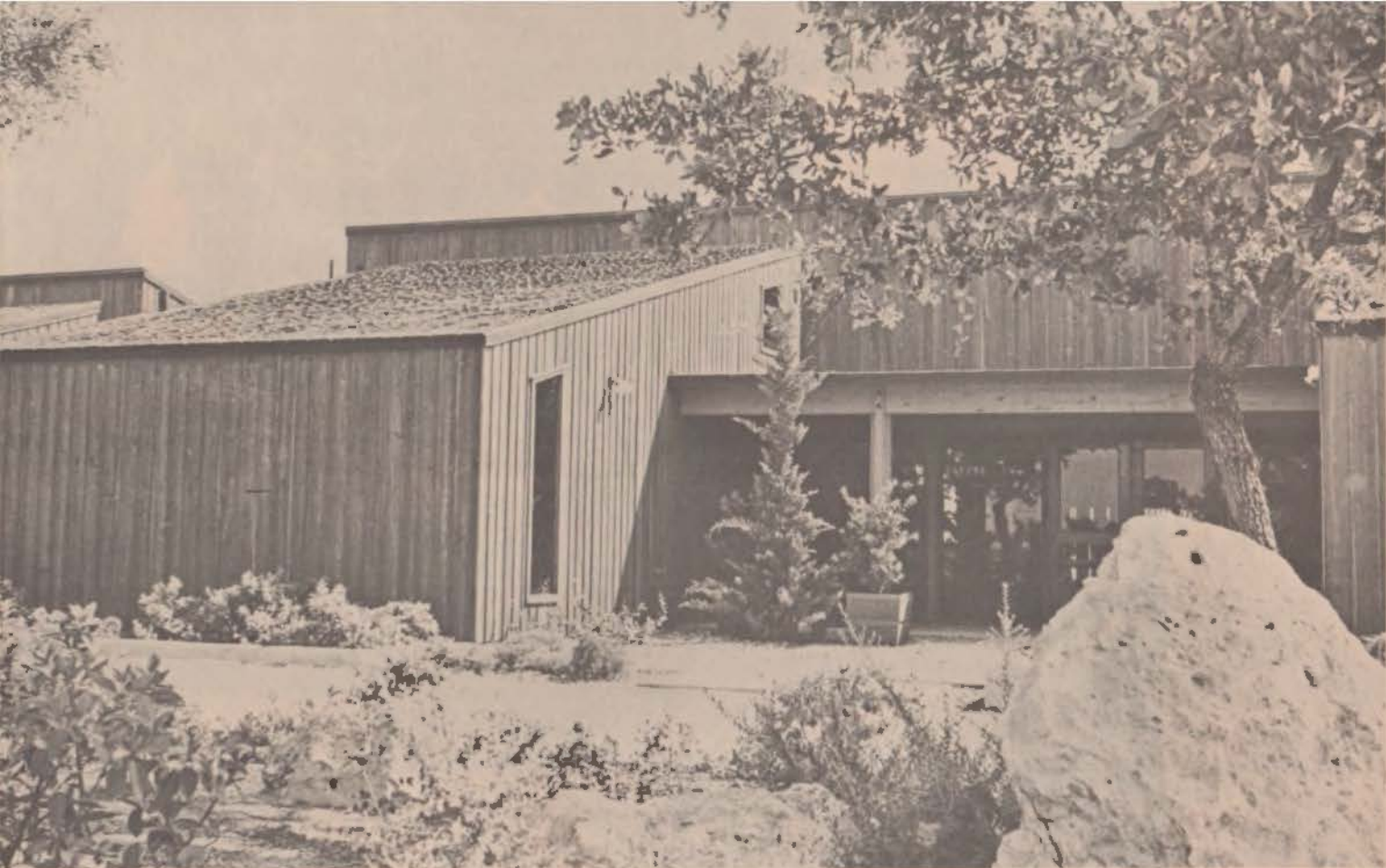
VIEW TOWARD ENTRANCE
