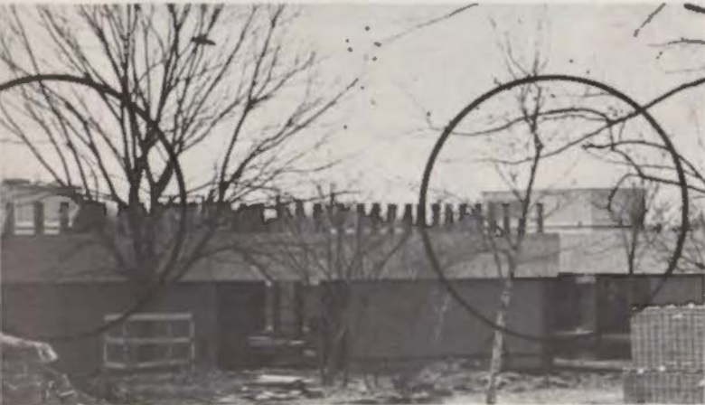
Subsystem No. 2 – HVAC-
