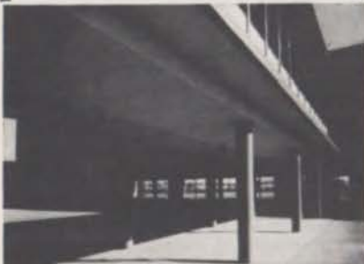
H. S. Thompson School, Dallas, Texas Architect: J. Allen Boyle Plaster Contractor: Storbeck & Gregory X-59 used in ceiling of ground floor.
