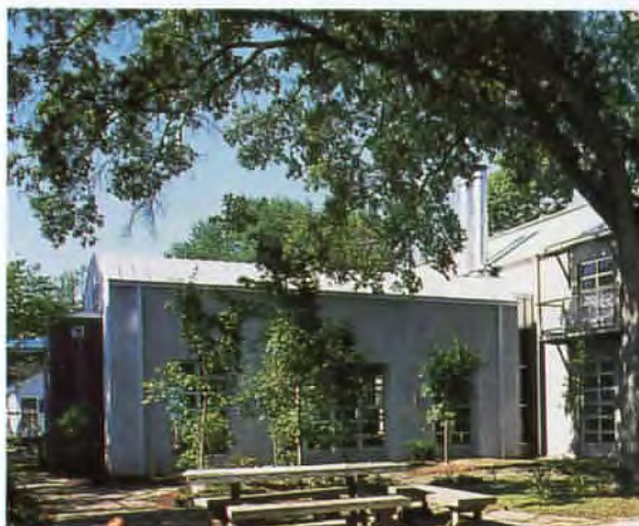
Above: The main two-story volume of the house is clad in concrete block; a metal-clad living and dining wing divides the lot's courtyard spaces.
