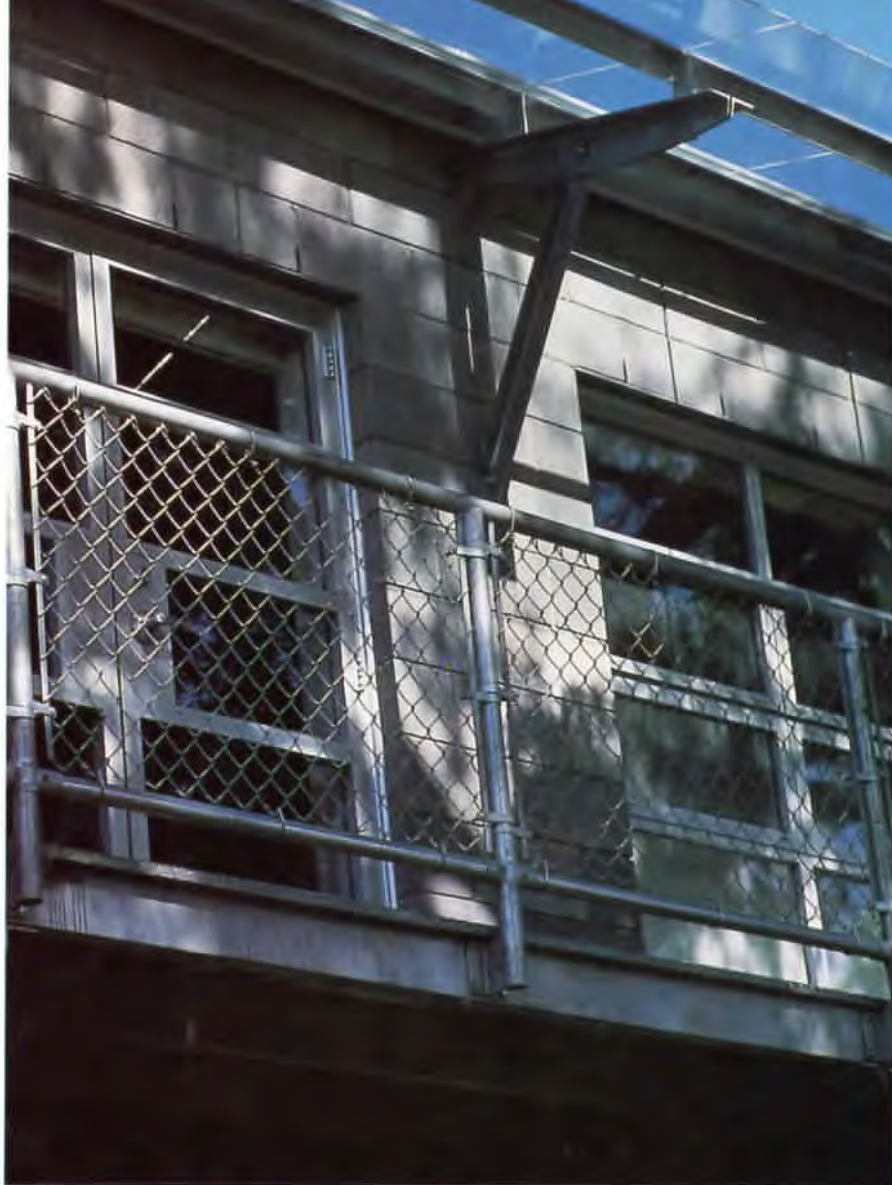
Above: The second-story sheltered walkway at Jaral, the residence in Houston by Taft Architects, is set in front of expanses of casement windows, evidence of the emphasis on natural ventilation throughout the house.
