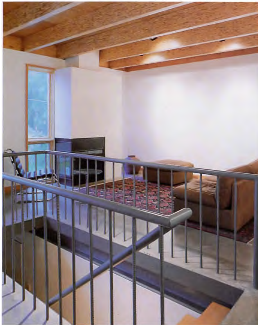
Above and right: Beams of laminated wood particles, concrete floors, and steel framing provide the character for the second-floor living-room area in Cunningham Architects's Travis Apartments.
