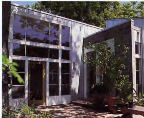
Far left: Plan; the house consists of two staggered 20-foot-wide metal sheds, one for the bedroom wing, the other for common areas. The wings also define protected outdoor spaces.
