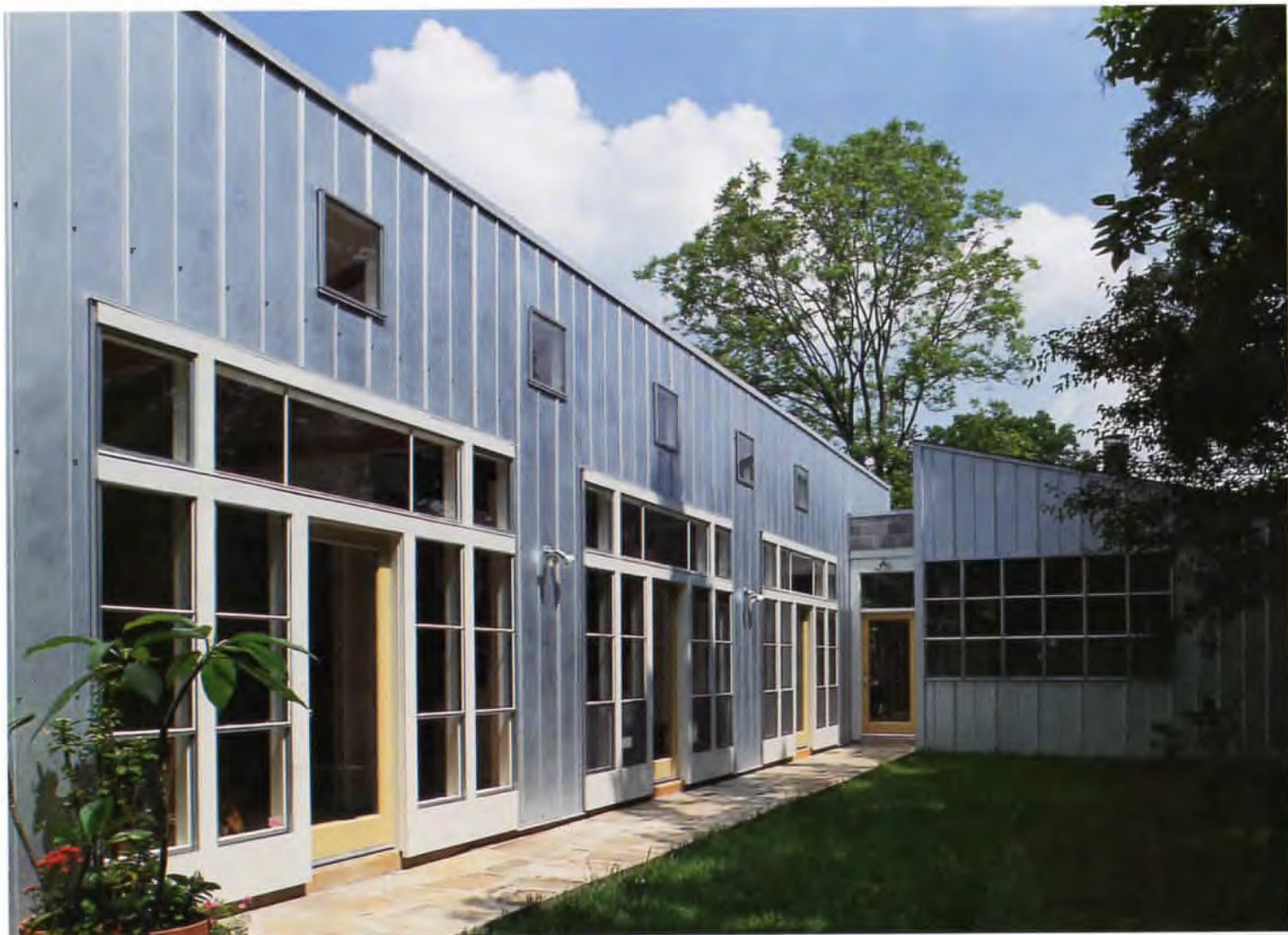
Top: The Balinskas House's interior gallery, which looks out onto the fenced-in sideyard, channels natural light into the bedrooms.
