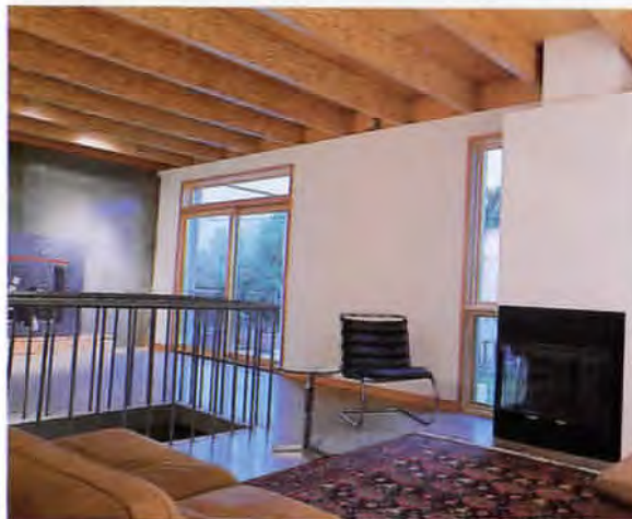
Above and right: Beams of laminated wood particles, concrete floors, and steel framing provide the character for the second-floor living-room area in Cunningham Architects's Travis Apartments.
