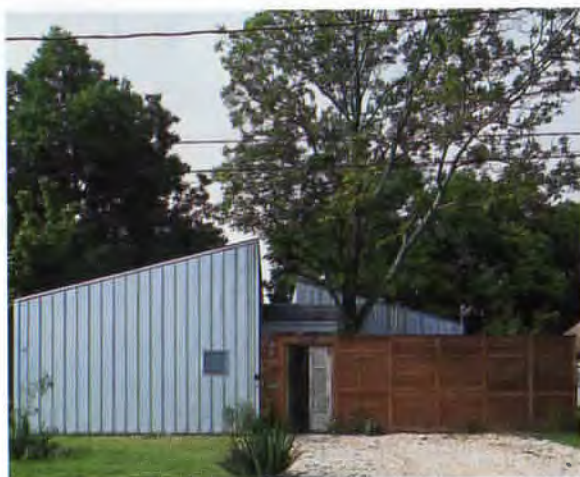
Right: The metal-sided living wing and an antique mesquite-wood gate form the entrance, which leads into the courtyard.
