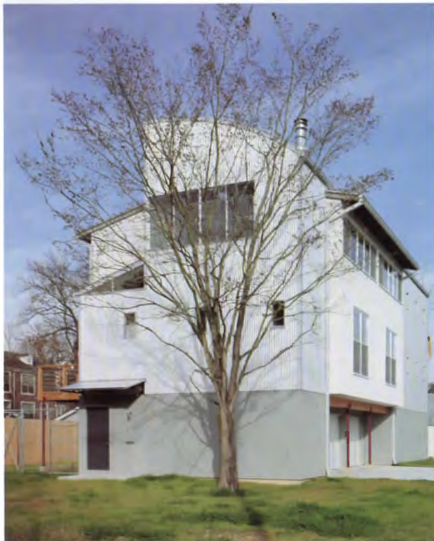
Above: The zones of the Bennett House + Studio in Houston by Val Glitsch, AIA, Architect are expressed in different forms, roof materials, and window systems.
