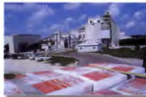
White Cement Plant, Waco, TX
