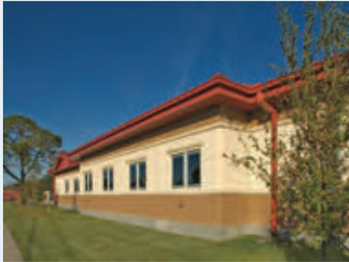
Fibrebond's innovative construction method uses **precast concrete** buildings to shorten the time from architectural design to project completion.
