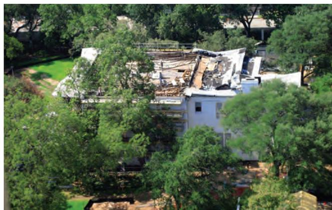
(left) A photo from November showed stabilization efforts that protected the 1856 mansion from the elements as work crews began to prepare for its eventual restoration. (above) The fire caused heavy damage to the attic and roof.
