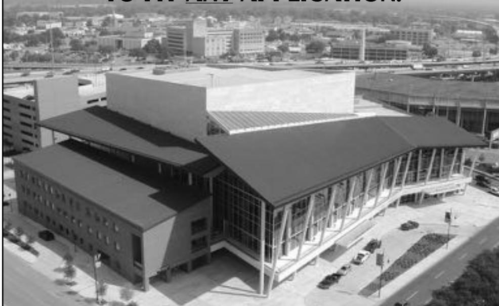
Berridge's Cee-Lock Standing Seam Roof System provides the distinctive finish to the angular, skewed roof shapes of the new Hobby Center for the Performing Arts in Houston. Berridge "Colonial Red" Kynar 500® finish contrasts dramatically with limestone, glass, and brick walls, and steel columns, as well as the urban surroundings.
