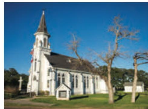
Cyril and Methodius Catholic Church. Characterized by the Carpenter Gothic style with tall, narrow, four-over-four, pointed-arch windows, the church is a basilican three-aisle plan. A steep gabled roof covers the rectangular volume
