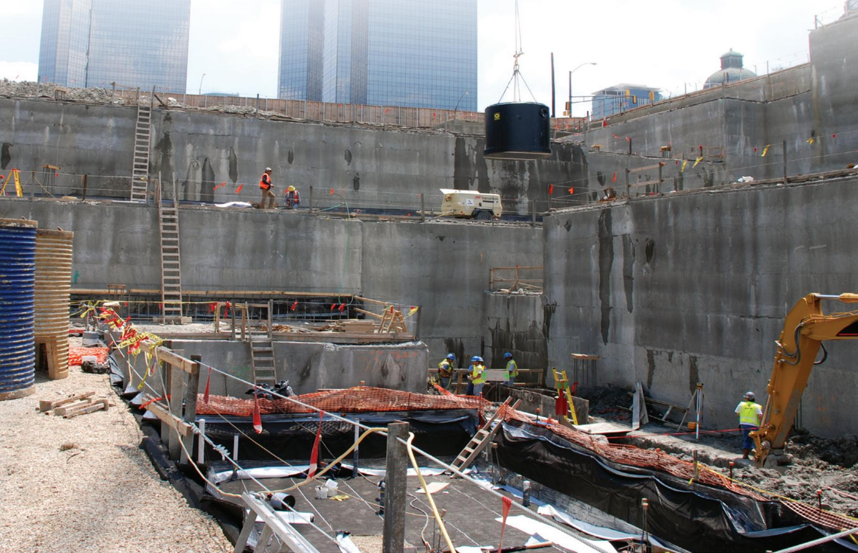
In building the Tarrant County College Trinity River East Campus in Fort Worth, Polyguard Underseal<sup>®</sup>, both Underslab and Blindside, was used as waterproofing. As you can see, lots of detailing was required. Detailed areas are where most leaks occur throughout the building envelope.
