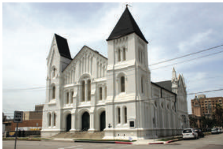
First Presbyterian Church, 1903 Church Street
