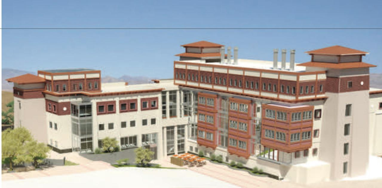
teams have also been requested to introduce different roof designs. The COHS/SON has integrated a *lung-go* roof system, essentially a stacked double-gable roof. In Bhutan these are separated by a simple structural system to create a void allowing hot air to rise and exit thus naturally ventilating the building. In the case of the new educational building, a mechanical penthouse will be located between the roofs with air intakes strategically located between the eaves.
