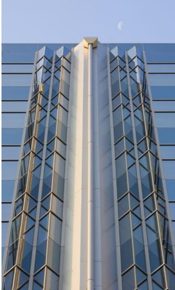
(preceding spread) The Margaret M. Alkek Building for Biomedical Research was completed in 2007. (this page, top) Lord Aeck & Sargent's architecturally expressed roof drainage system is integrated into metal columns. (this page, bottom) The metal armature casework systems provide visual lightness and functional flexibility to lab arrangements.
