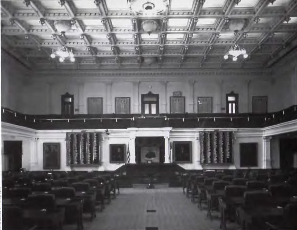
3 The House Chamber features a new audio system wired to each seat, a restored ceiling, and glass skylight. Air conditioning is supplied through the ventilator dome above each light fixture.
