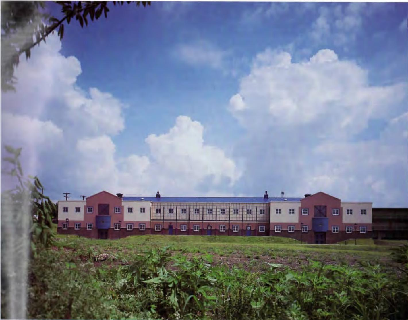
Loma Park elevation: Stucco, concrete block, tile, steel, and glass are combined in a landmark image.
