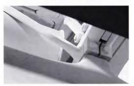
A crucial detail: the air-conditioning return-air duct tucked up above the leaves, under the glass. It removes heat before it gets down into the space below, but raises questions about the appropriateness of a glass roof for this type of building.
