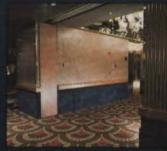
Matching pocket cover doors completely hide fire doors from view. Doors operate automatically on back-up DC power supply and are activated by any standard smoke alarm.
