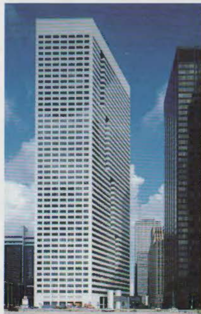
First City Tower, Morris*Aubry Architects, 1981. A parallelogram with stair-stepping vertical notches.
