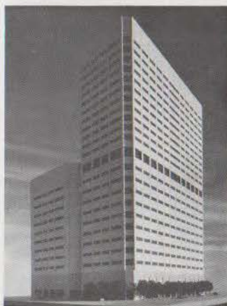
First City National Bank Operations Center, Houston, 25 stories, 1983. Morris* Aubry Architects, Houston.
