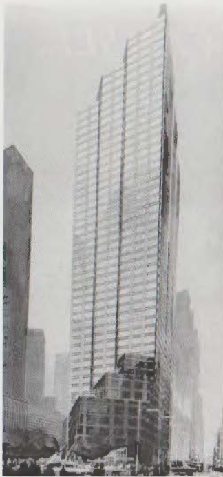
First City Center, Dallas, 50 stories, 1984. WZMH Group, Inc., Dallas.
