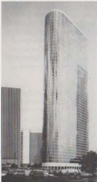
Four Allen Center, Houston, 50 stories, 1984. Lloyd Jones Brewer Associates, Houston.
