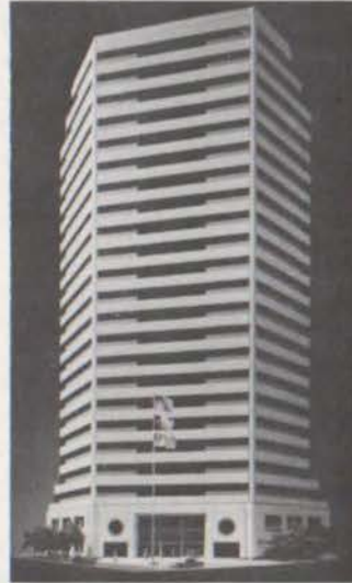
Texas Commerce Plaza, Corpus Christi, 23 stories, 1983. Morris* Aubry Architects, Houston.
