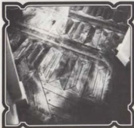
been taken from very old houses in Houston to rebuild the gables. These thin bevelled boards had many coats of paint and had to be stripped with corn starch, lye and water."
