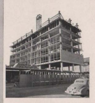
Upper photo shows 12-story section of Simms Building above the roof of block-square first flaor. The floors throughout are 6-in. thick reinforced concrete using a wide beam design and cantilevered 5 ft. outside the supporting columns. Architects and engineers: Flatow-Jason Moore. Contractor: Lembke, Clough & King, Inc. Both of Albuquerque.
