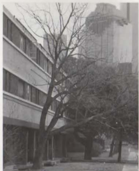
1 Allen Parkway Village, a public-housing project in Houston, sits in the shadow of downtown; a recent agreement may lead to the demolition of most of the project.
