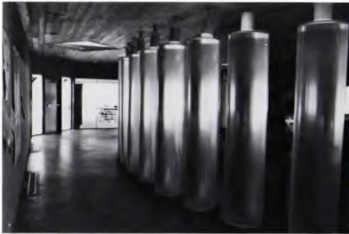
Water-filled plastic tubes retain heat from lights.
