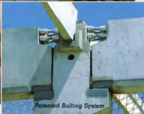
Amega is a general contractor that manufactures and erects precast, prestressed concrete buildings.
