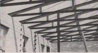
Stran-Steel trusses form clear-span roof over load-bearing masonry walls. Collateral material can be nailed to the steel!
