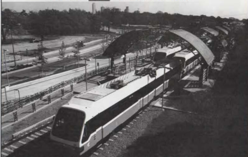
OPPOSING ARCHES FORMED BY BERRIDGE CURVED TEE-PANEL ROOFS ACCOMMODATE HIGH-VOLTAGE LINES FOR ELECTRIC-POWERED D.A.R.T. LIGHT RAIL TRAINS, VIA A CENTER OPENING
