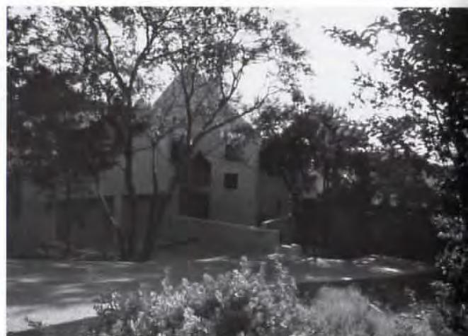
siphon" built into the stair tower at the entry takes advantage of prevailing summer breeze, while the use of solar shading from surrounding trees also contrib-
