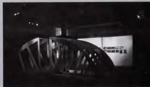
**The forms used to construct the Kimbell Museum's vaulted concrete**
