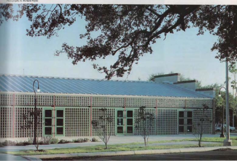
RIGHT: Inside the congregation area, the structure of the preengineered building is clearly visible, as is the exposed insulation system of batt panels held with painted chicken wire. BELOW: Along the street facade, the only symbol of the building's religious function is quatrefoil glass block above each bay.
