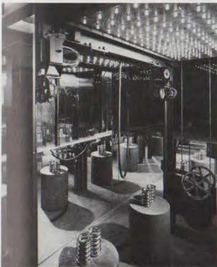
Underside of elevator and mirror-clad pit; chrome springs and gear wheels.
