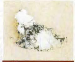
EIFS damaged by hail in Fort Worth.
