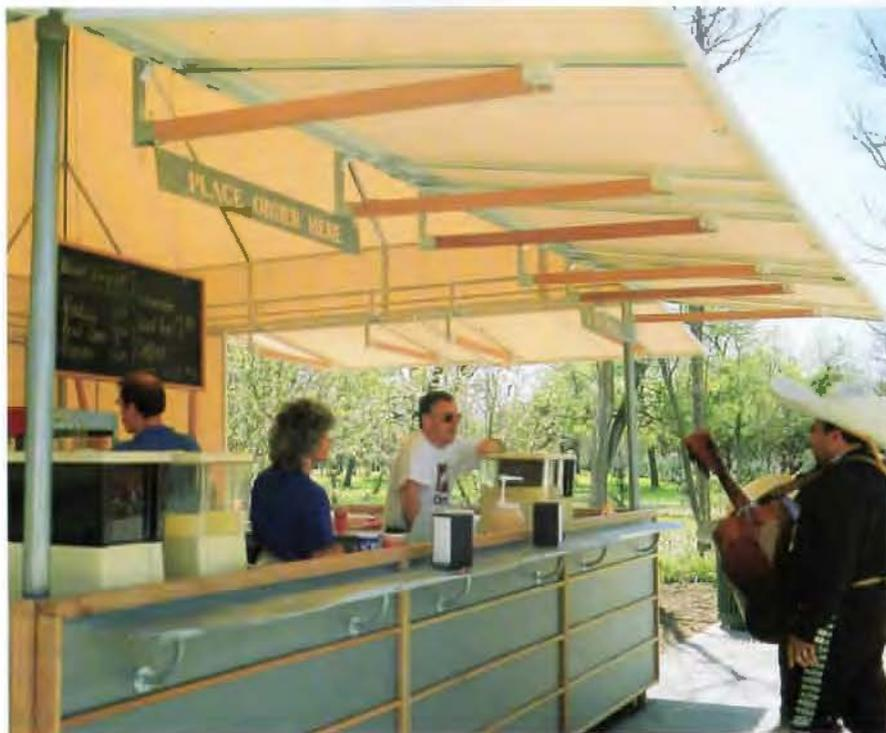
**Below: Cabinets on casters form the stand's walls, while canvas flaps are raised on welded brackets to form awnings for the serving area.**
