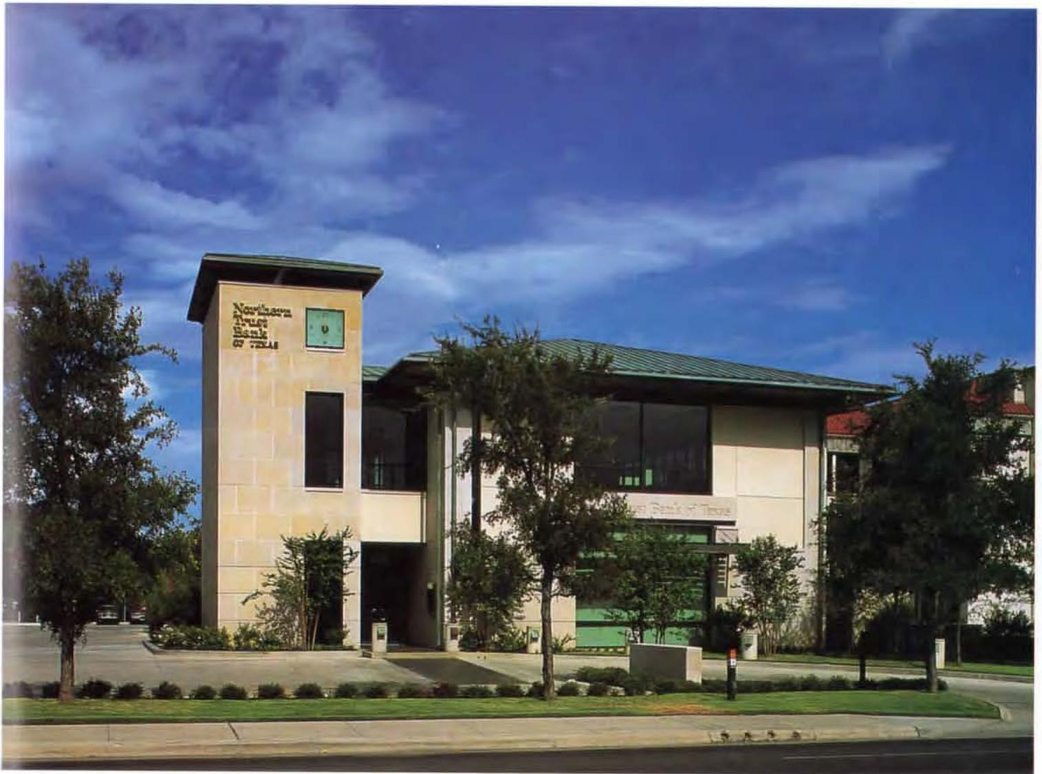
**Facing page, top:** Wide eaves with stained-cedar soffits are held on tapering steel brackets, while copper gutters and painted window frames bring contrasting color to a cleanly detailed limestone wall; a steel-columned pergola shades a walkway.
