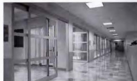
**FireLite**, a clear, wireless ceramic glass, looks and cuts like real glass. Distributed by **Technical Glass Products**, FireLite can be installed in standard fire-rated frames. Listed by Underwriters Laboratories and Warnock Hersey International, FireLite carries a fire-rating of 60 minutes in sizes to 1,296 square inches and 90 minutes in sizes to 100 square inches.
