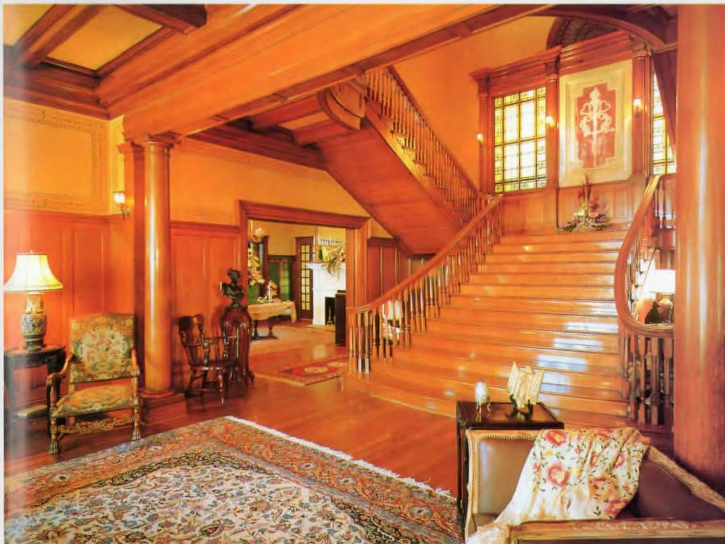
**Above:** The grand stairs, with their double-cantilevered landings, were visibly sagging when the restoration process began. At the top of the stairs, the long clear span was reached and restructured from the attic floor above, thus preserving the free-hand oil painting on the plaster coves.
