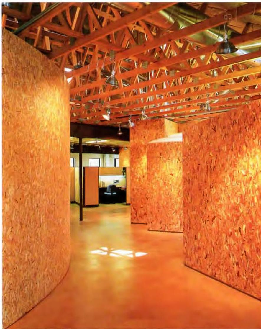
**Above: The World Neighbors headquarters was built on a budget of less than \$20 per square foot by emphasizing such materials as concrete, corrugated fiberglass panels, and oriented-strand-board walls.**
