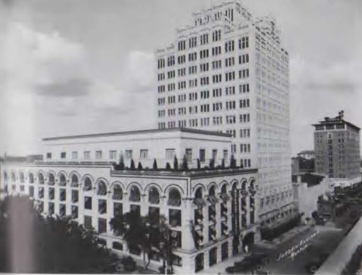
TSA offices occupy stepped-back floor at top of Norwood Tower, shown here in an early photograph along with its connected parking garage. The garage's elaborate fenestration was lost to modernization in the 1950s.
