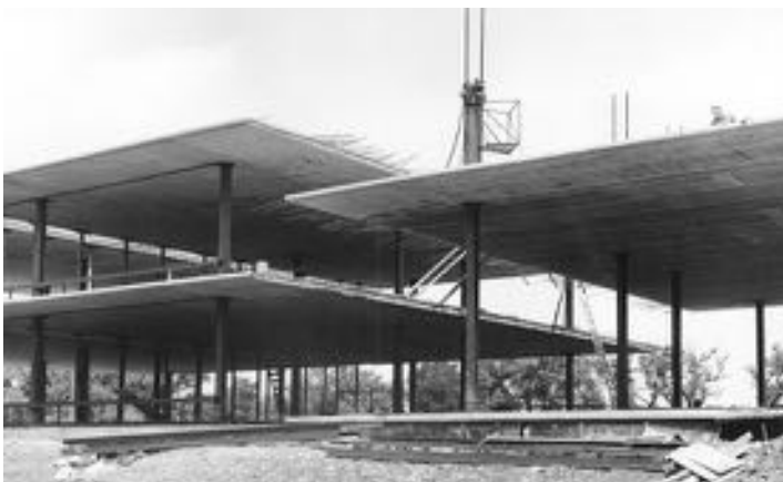
(top) The Youtz-Slick Lift-Slab technique employed in building Northrup Hall was its first use in a major construction project; courtesy Alexander Architectural Archive. (bottom) The replacement Northrup Hall will be a new focal point for the campus; rendering by Thomas Schaller for Robert A.M. Stern Architects.
